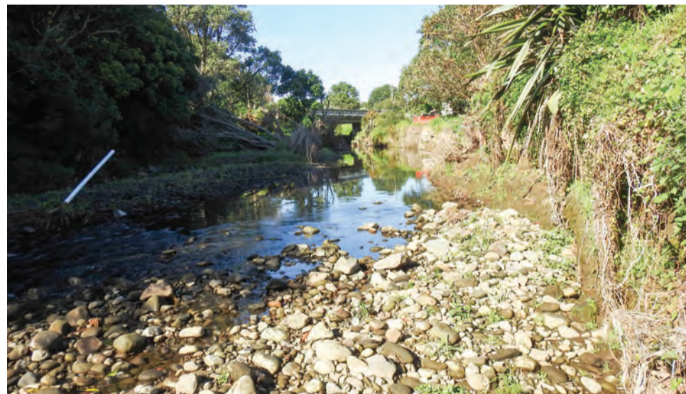
A section of the walkway downstream from the Otahi Bridge was washed out.
