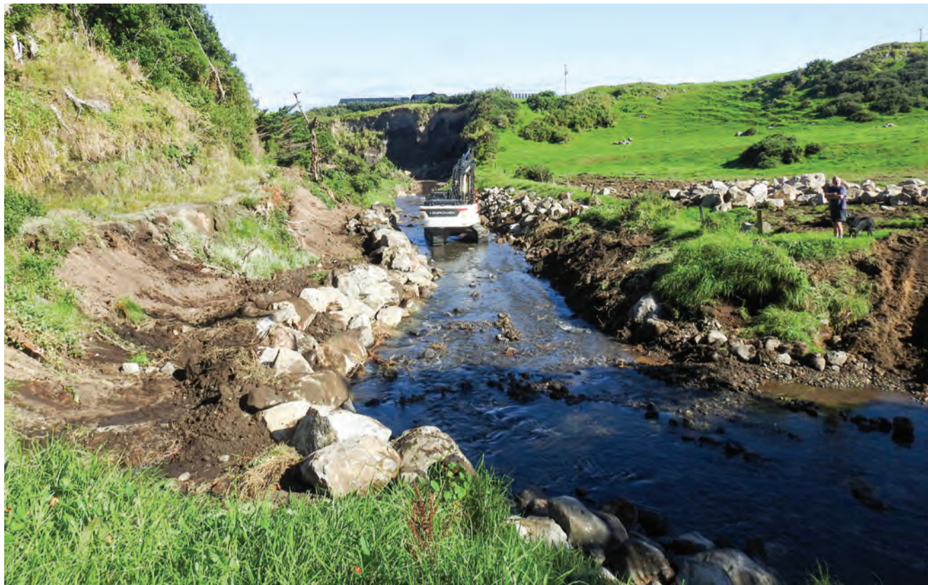
Gibson Contracting's 35 ton digger working away at the Otahi Stream.
